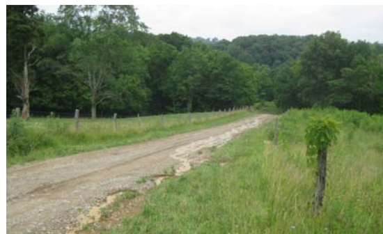
Runoff from the road surface during a natural rain event at the study location.
